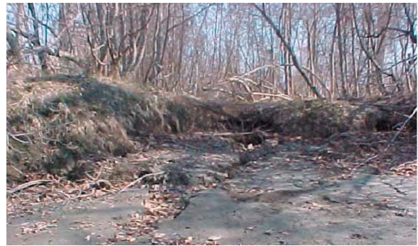
If undesirable conditions like stream bank erosion are identified, management actions may be implemented
