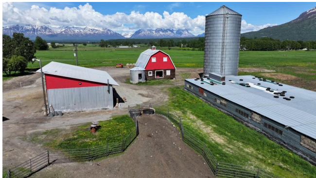
Attachment 3: The barn after the DePriest family replaced the rotting logs at the base of the barn and restored the red paint.
