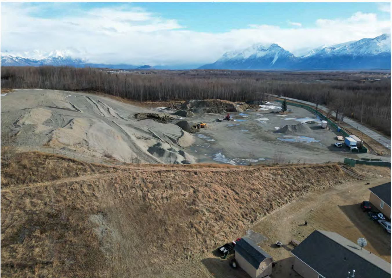
Aerial view to east of Phase 1. Earth berm behind residential structure providing noise and visual abatement.
