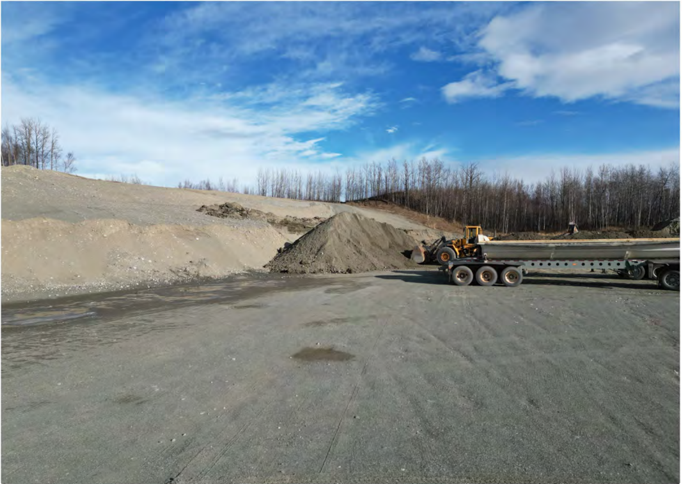
View to east, pit floor in foreground, working face serves as visual and noise barriers thru phasing.
