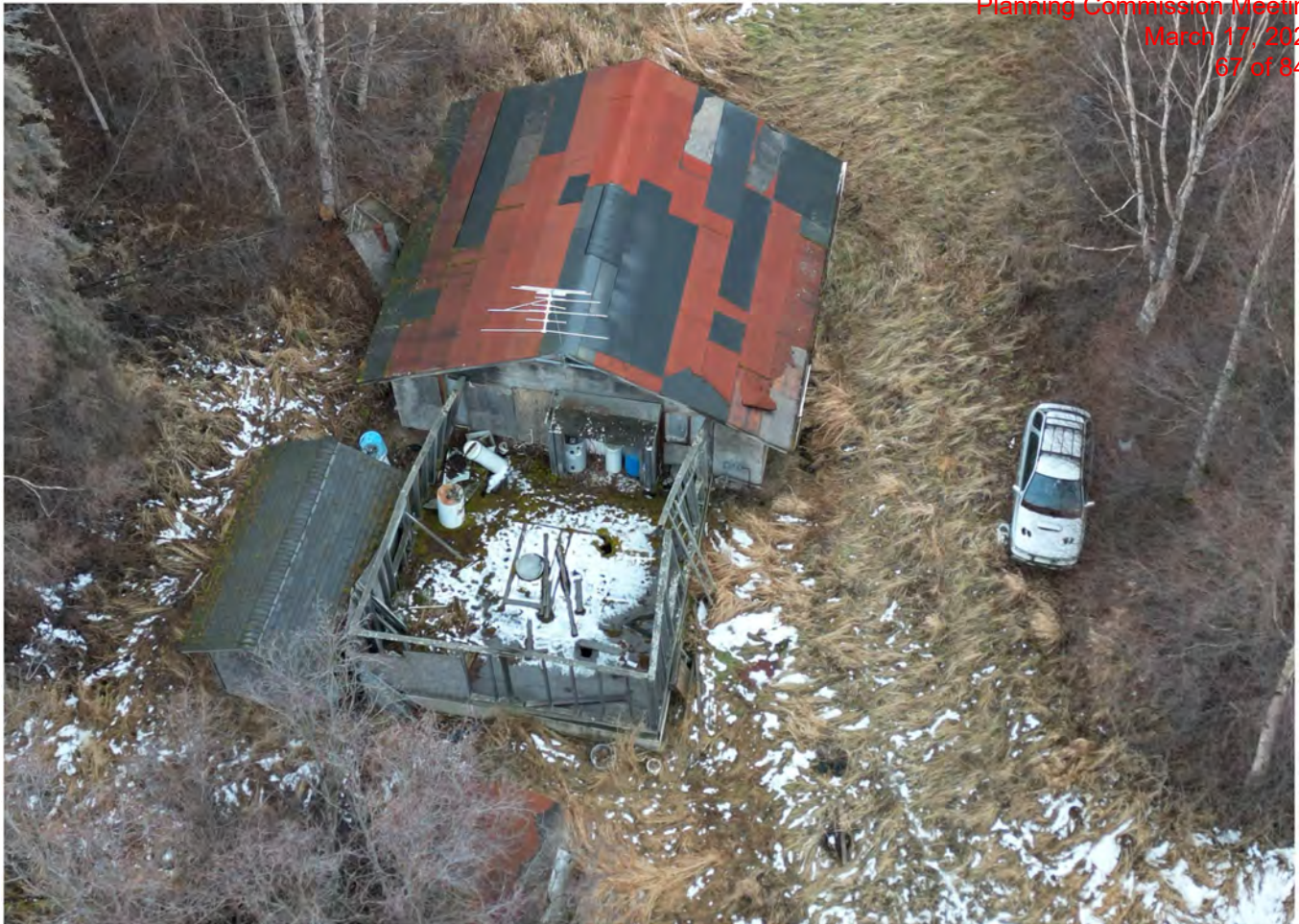
Aerial view of derelict residential structure on subject property. View towards southeast.
