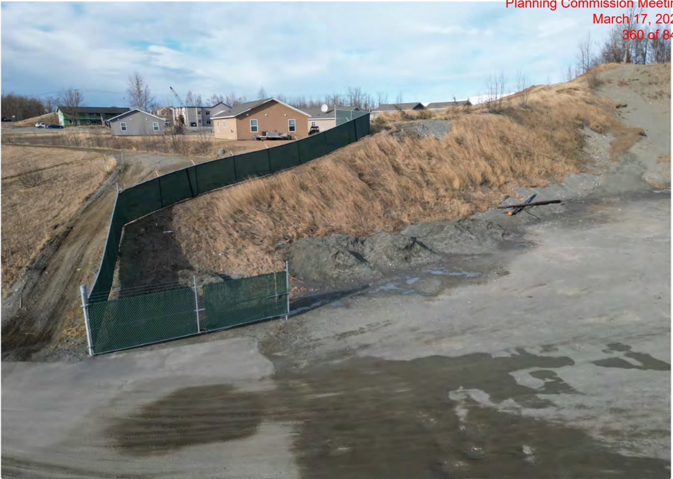
Aerial view to west, earth berm and fence slating serving visual and noise abatement (center photo).
