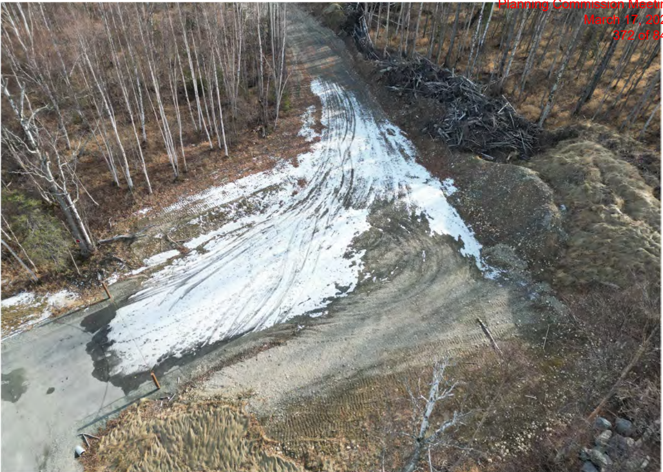
Aerial view of pending driveway access at E Brenda Ave. Not for hauling earth material. Secured by chain and lock.
