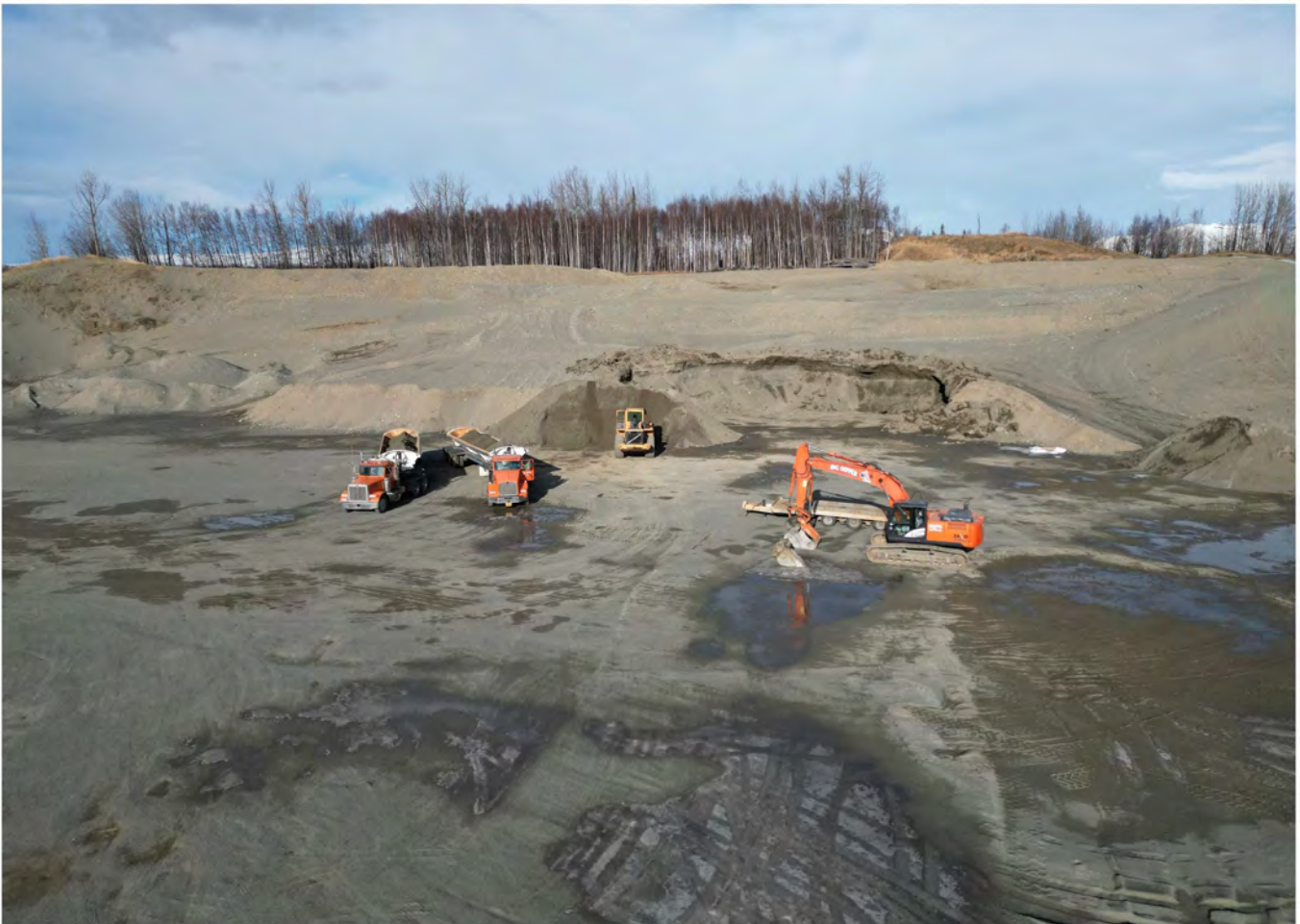
Aerial view to north from Tract 2. Working face of Phase 1, operational area, and pit floor depicted.
