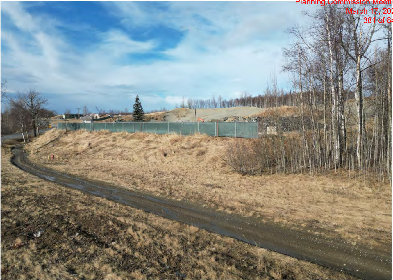
Aerial view to northwest, cloth screen on fencing for visual abatement to East Fairview Loop. Photo taken over Fairview Lp.
