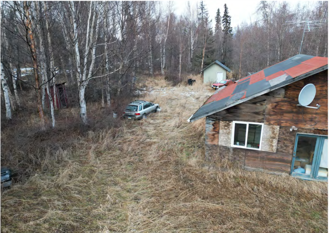
Aerial view of derelict residential structure and junk vehicle on subject property. View towards north.
