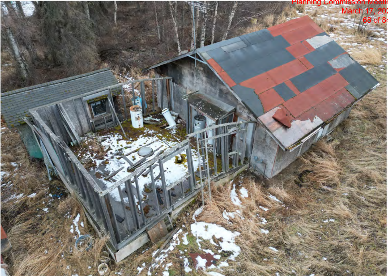
Aerial view of derelict residential structure on subject property. View towards southeast.
