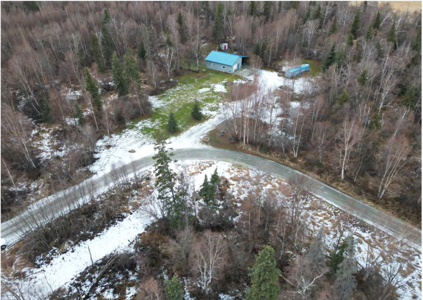
Aerial view northwest over proposed tower site at approx 155'. S Lindsey Circle & adjacent residential structure pictured.
