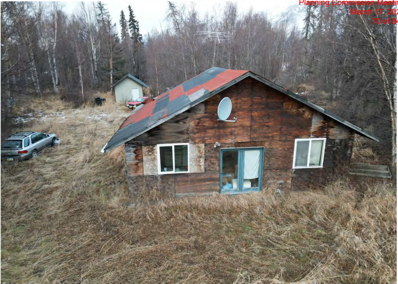
Aerial view of derelict residential structure and junk vehicle on subject property. View towards north.
