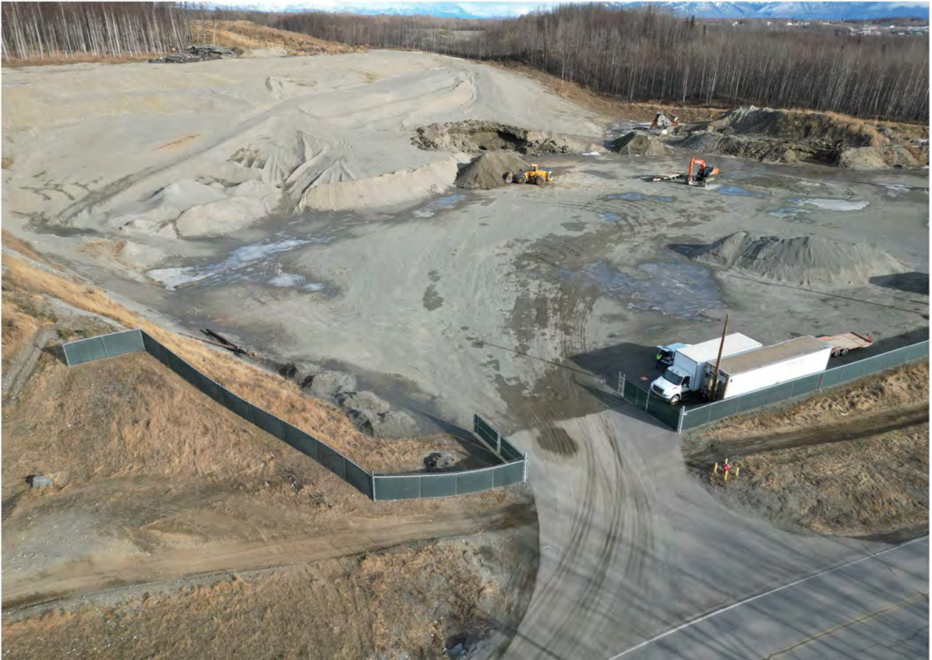
Aerial view to northeast of Phase 1.
