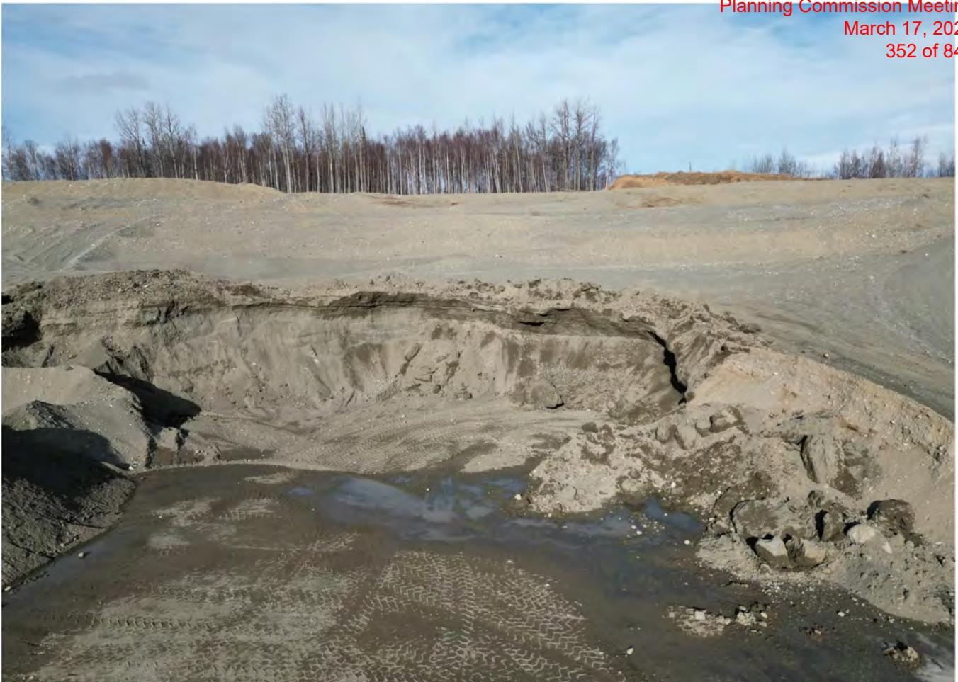
View to north, working face of Phase 1 providing visual and noise abatement to neighboring uses.
