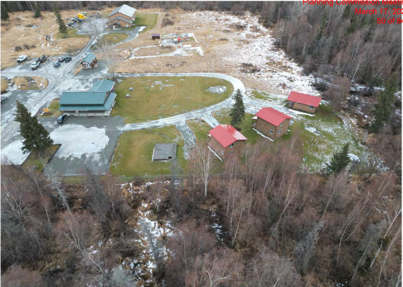
Aerial view east over proposed tower site at approx 155'. Pics of commercial structures w/ unregistered helipad (top center)
