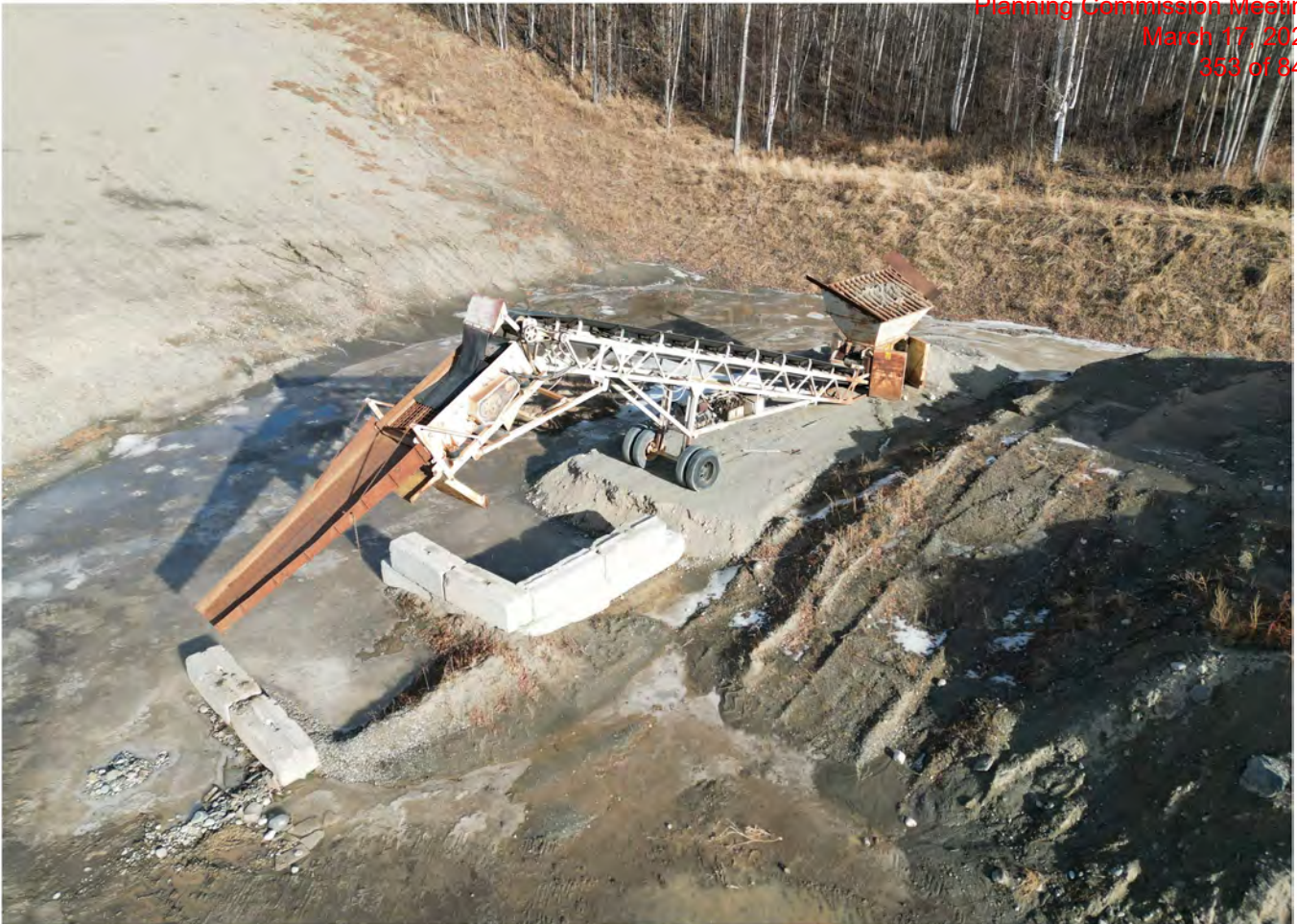
Northeast aerial view of mobile material screener
