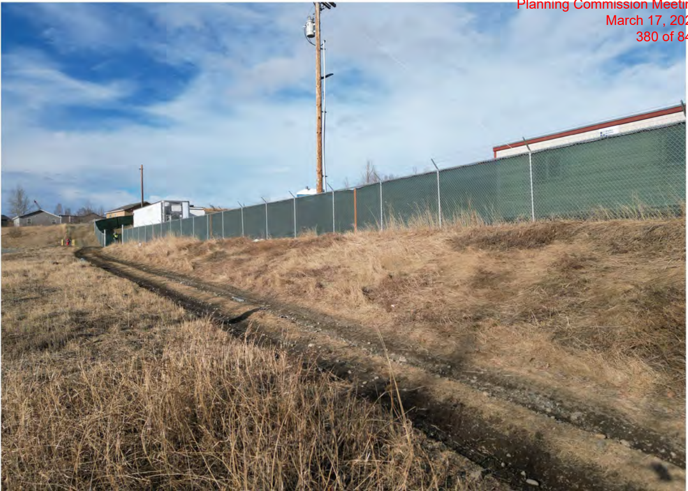
View to northwest from E Fairview Lp with pit entrance pictured left. Cloth screen for visual abatement to roadway.
