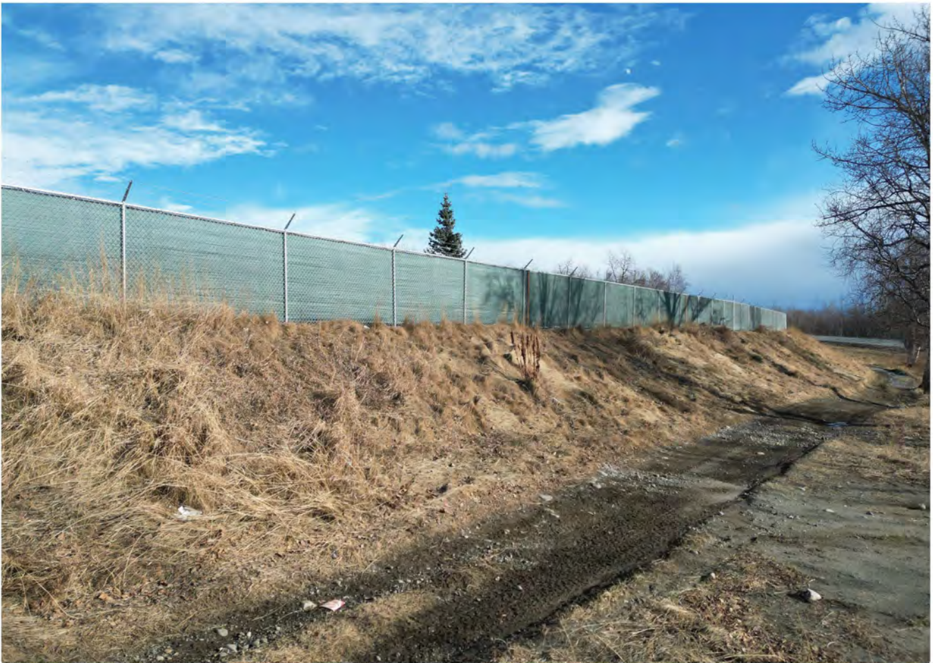
View to east from E Fairview Lp. Cloth screen for visual abatement to roadway.
