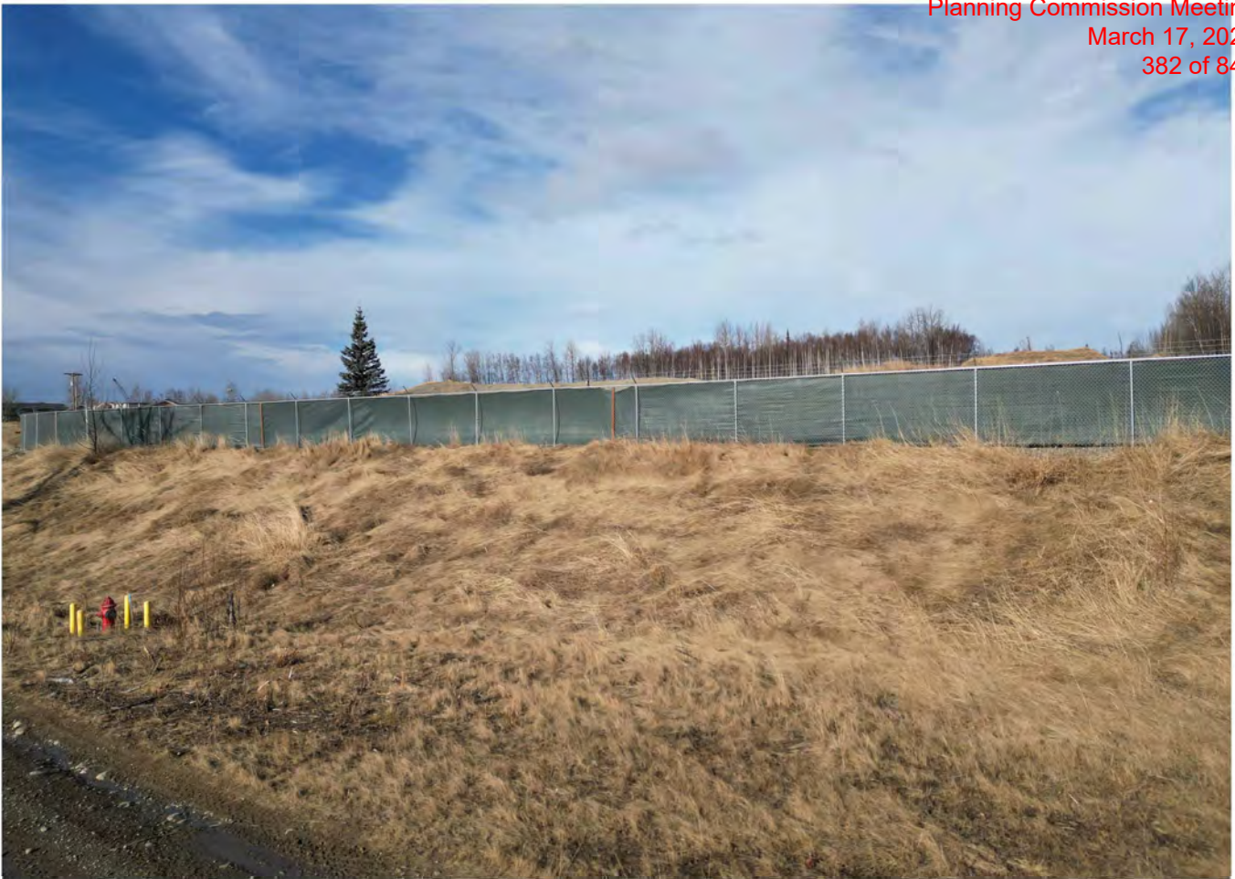
Aerial view to north, cloth screen on fencing for visual abatement to East Fairview Loop. Photo taken from E Fairview Lp.
