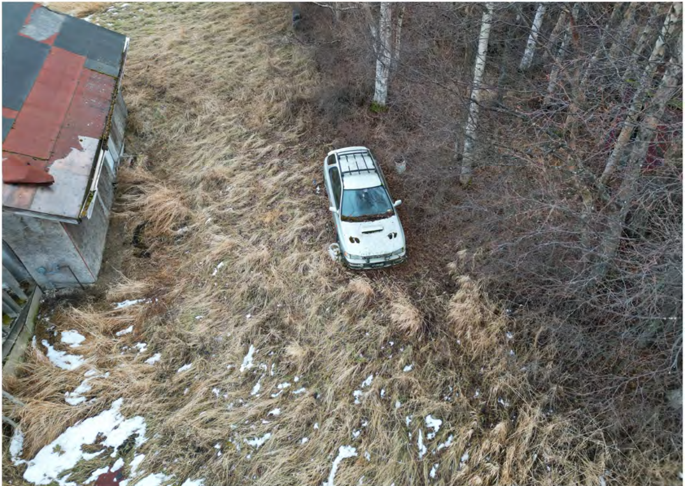
Aerial view of derelict residential structure and junk vehicle on subject property. View towards south.
