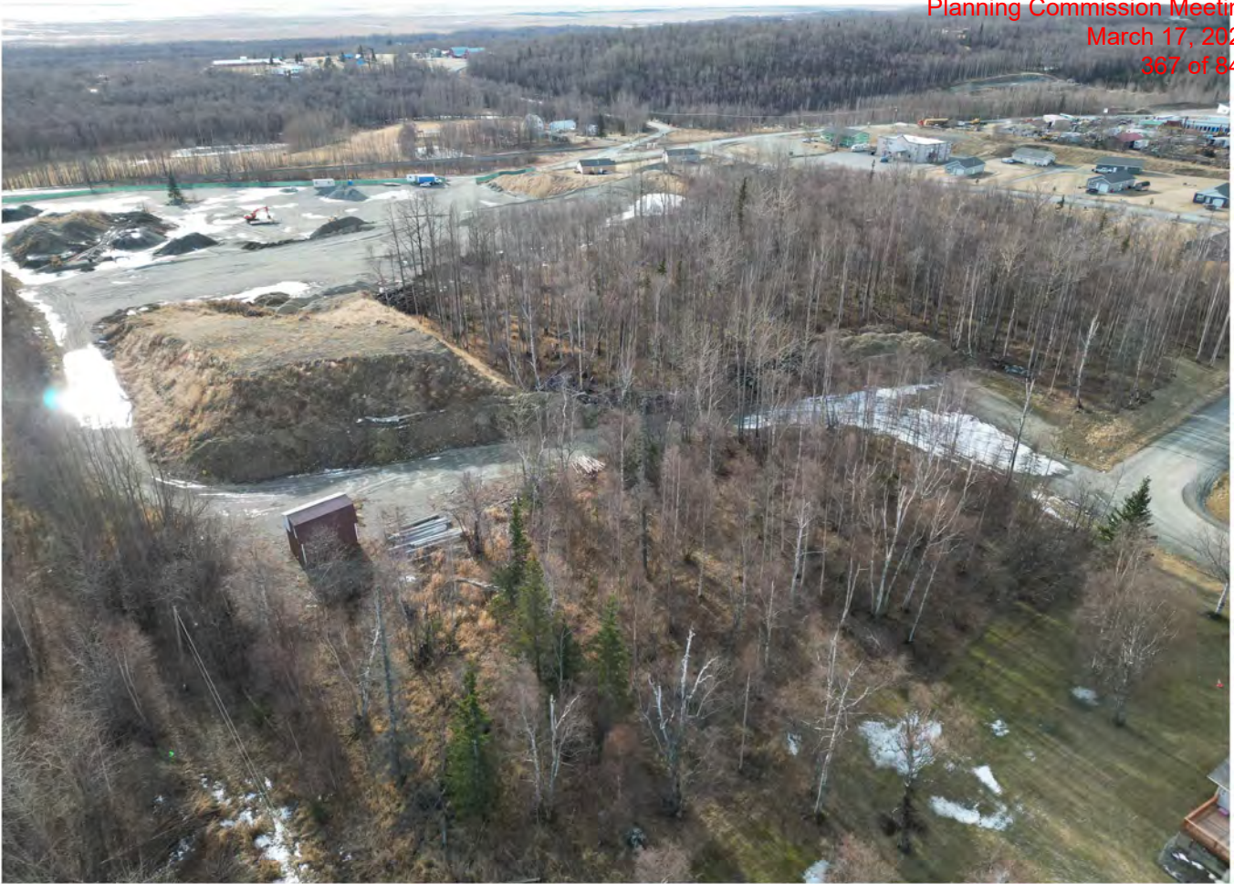
Aerial view to southwest, Tract 1 (bottom right), Tract 2 (top/left). Internal driveway away from adjacent residential uses.
