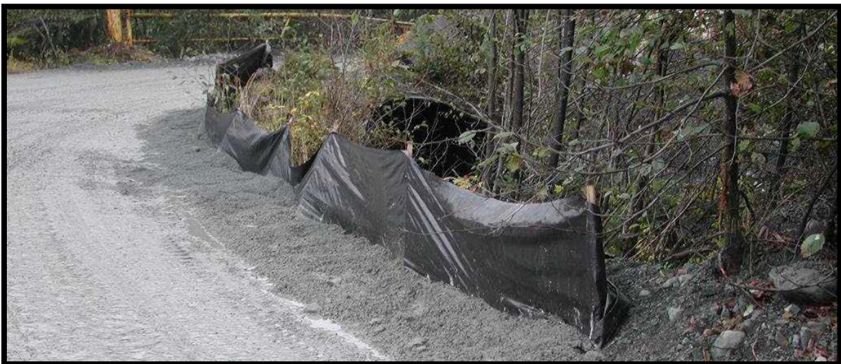
Figure 7-8: Silt Fence Example (Photo: City and Borough of Sitka)
