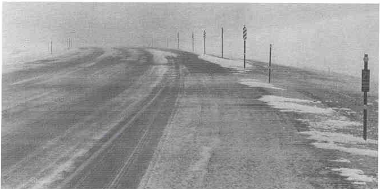
Figure 3. Improved visibility downwind of a 12-ft. (3.7-m) snow fence. The top photograph was shot 200 ft. (60 m) outside of the protected area. The bottom photograph was taken at the boundary of the protected area. (Photographs by Keith Rounds, Wyoming Department of Transportation.)
