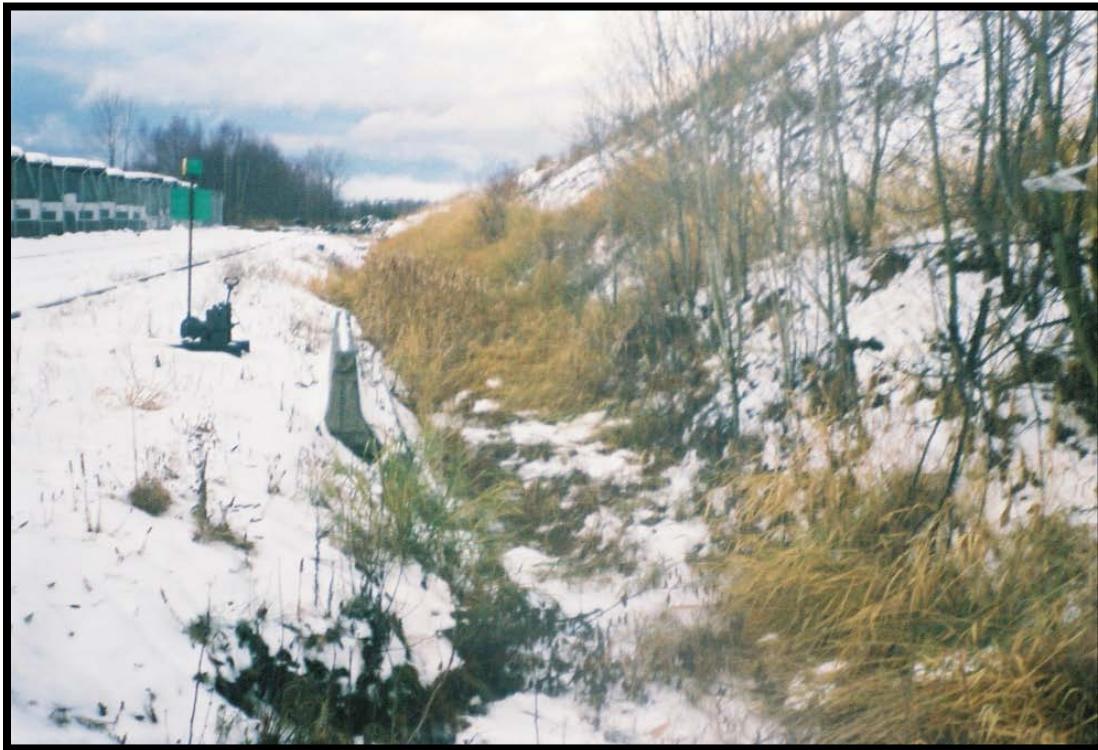
Figure 7-12: Ditch Example (Photo by permission of Central Paving Products, Anchorage Alaska)
