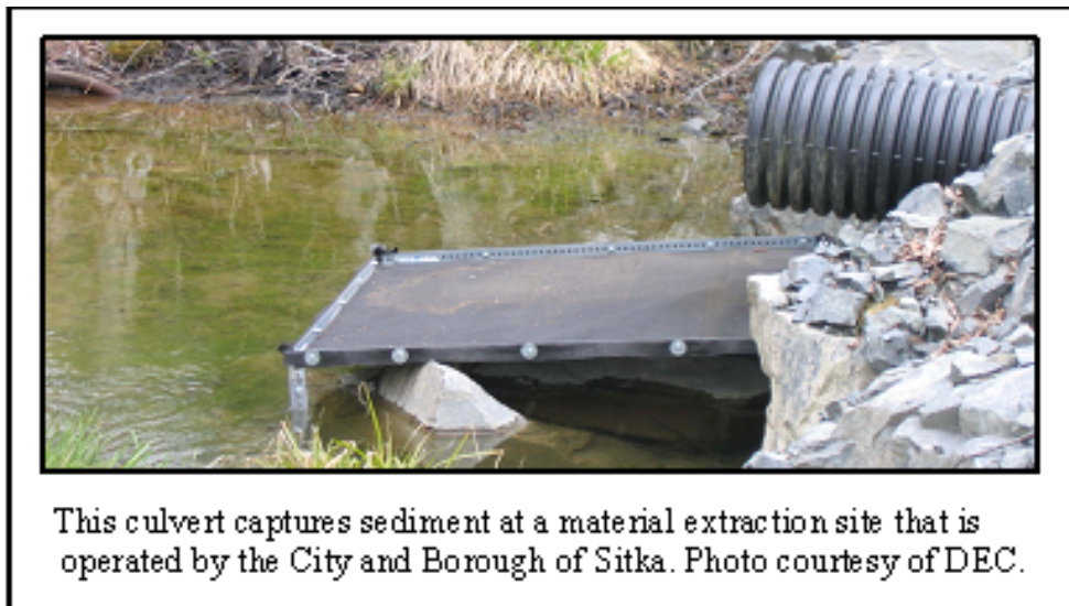
Figure 7-5: Outlet Protection Example
