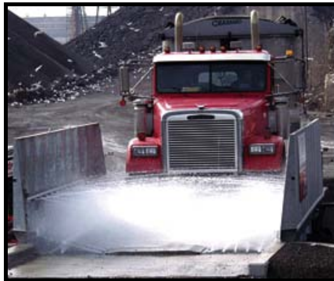
Figure 8-5: Wheel Washer with Sprayers (Photo from January-February issue of Erosion Control Magazine article “Controlling Fugitive Dust on Roadways” by Carol Brzozowski)
