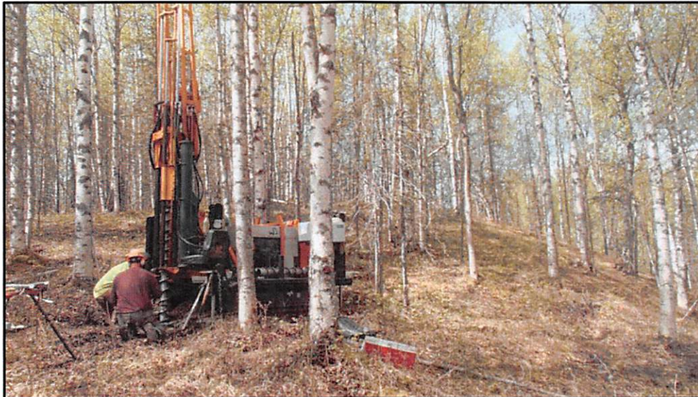
Note: Drill rig positioned at Test Boring RM23-05, 26 May 2023.
