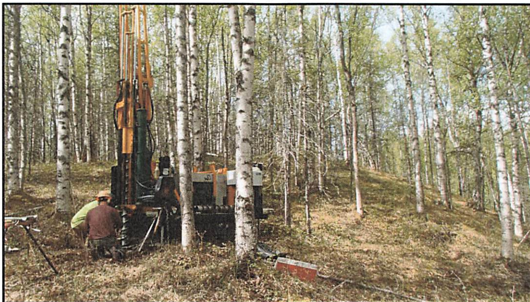
Figure 1. CME-55 Drilling Rig on Tracked Carrier
