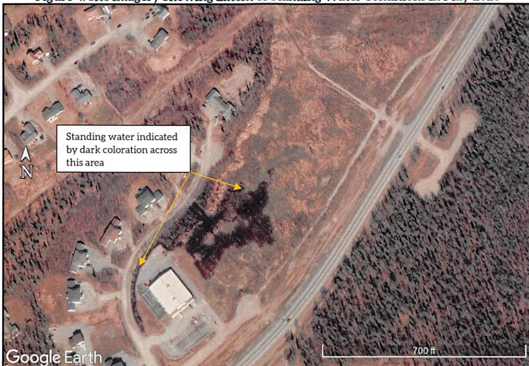
Figure 4: Site Imagery Showing Extent of Standing Water Conditions in May 2020
