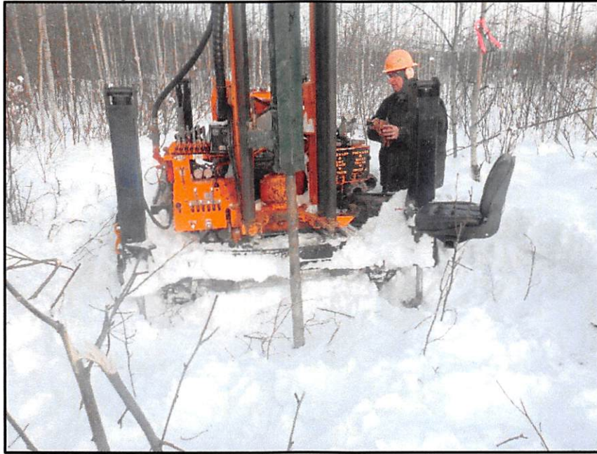
Figure 2: CME-55 Drilling Rig on Proposed Lot 1A
