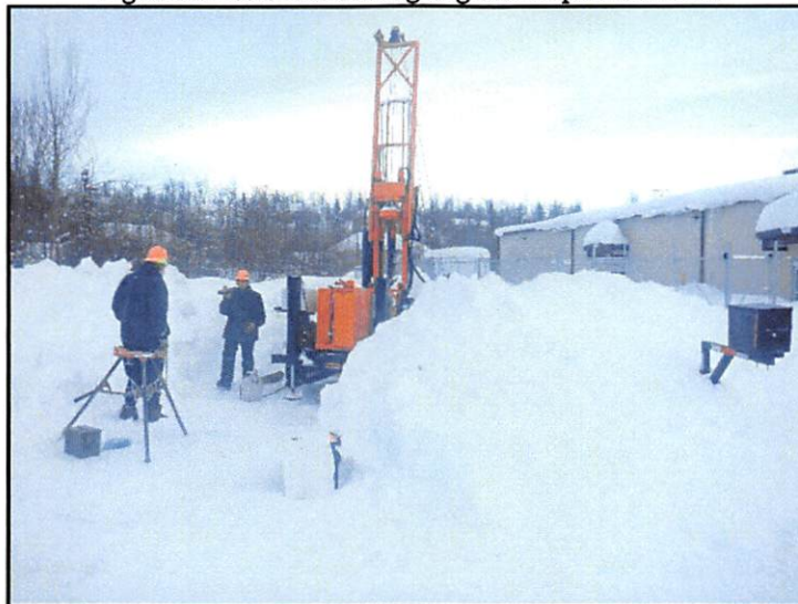
Figure 1: CME-55 Drilling Rig on Proposed Lot 1B
