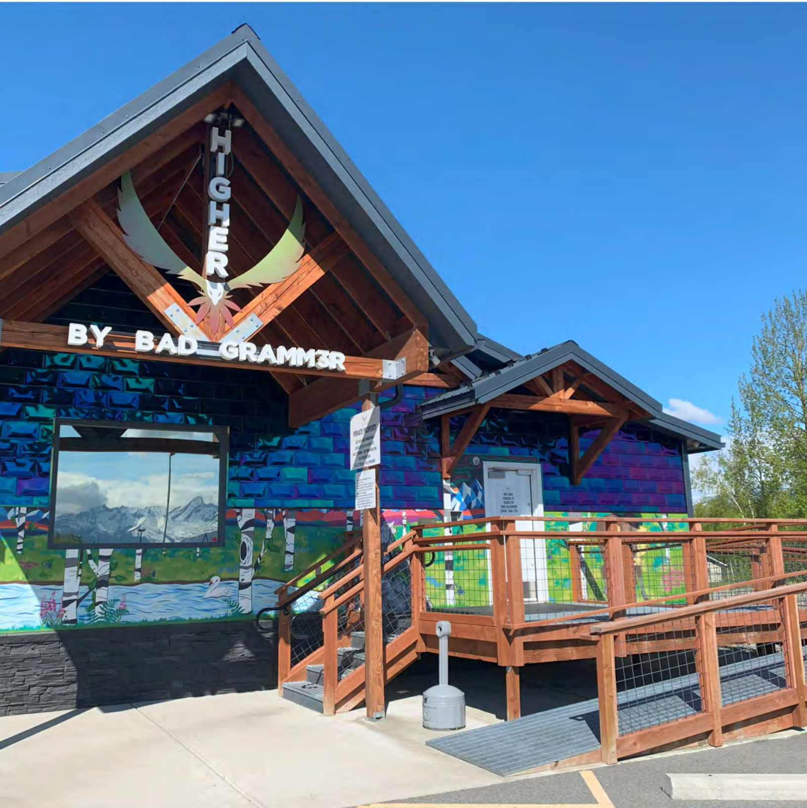
Existing Retail Facility to be moved
