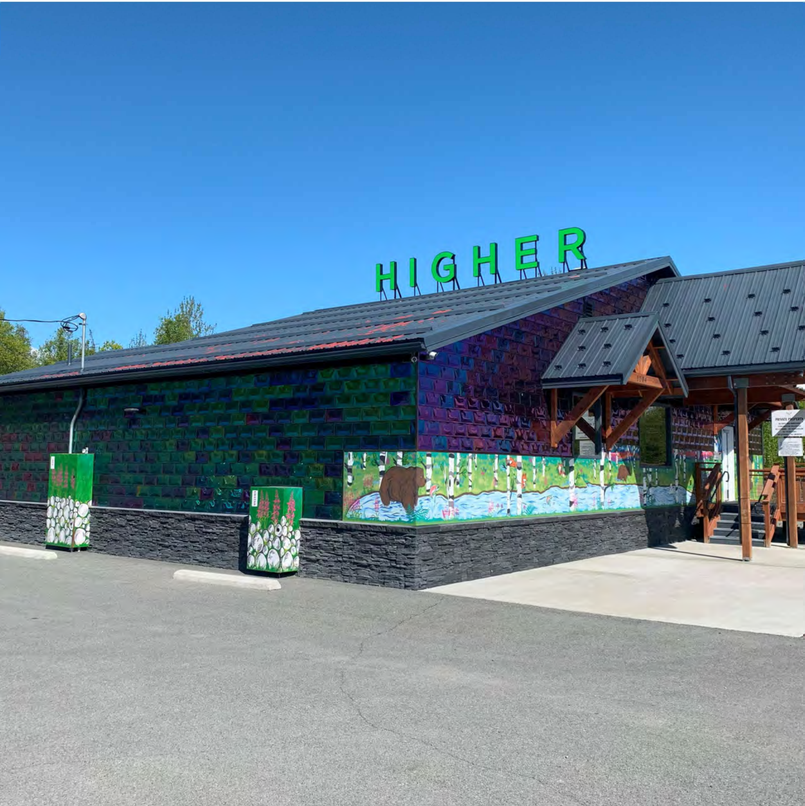
Existing Retail Facility to be moved
