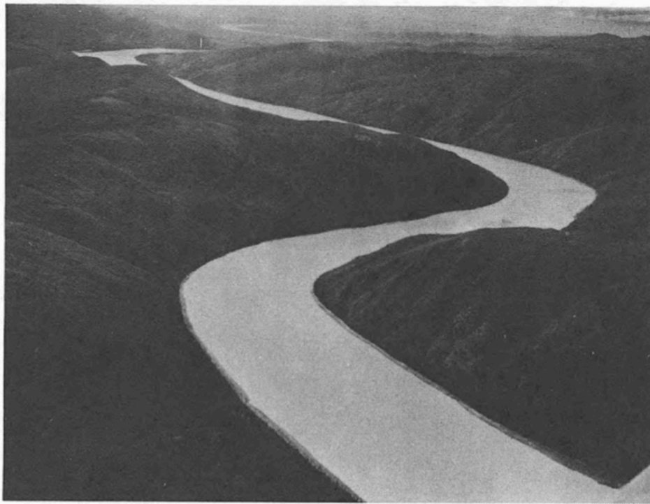
Figure 5. Preferred "Denali" location for the 1950s upper dam, located about 115 miles upstream of Devil's Canyon. From USACE 1975.
