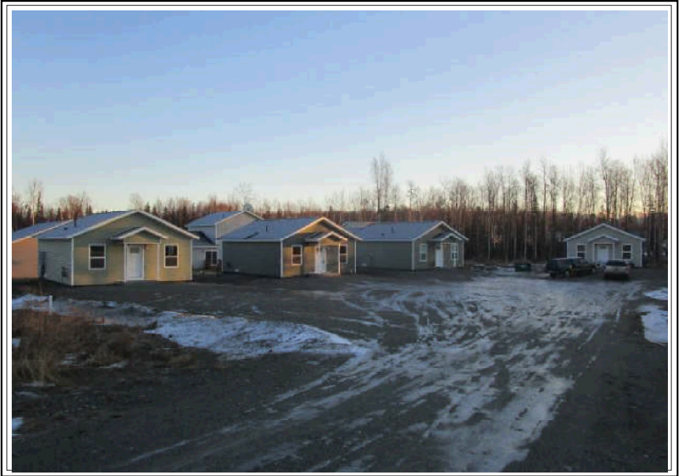
FRONT VIEW OF SUBJECT PROPERTY
