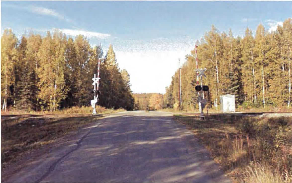
Figure 14. Cheri Lake Drive at-grade Railroad Crossing
