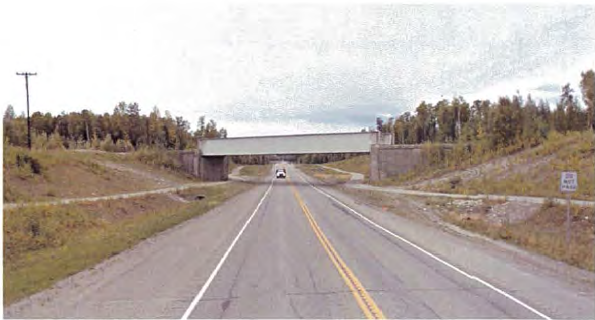
Figure 13. Alaska Railroad Separated Grade Crossing of the Parks Highway
