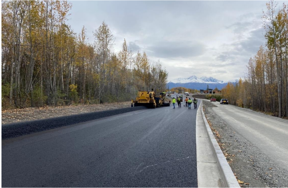
Above photo: Felton Street Mainline Paving
