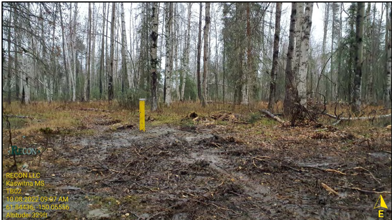
Figure 7. TB02 - Typical monitoring well installation.
