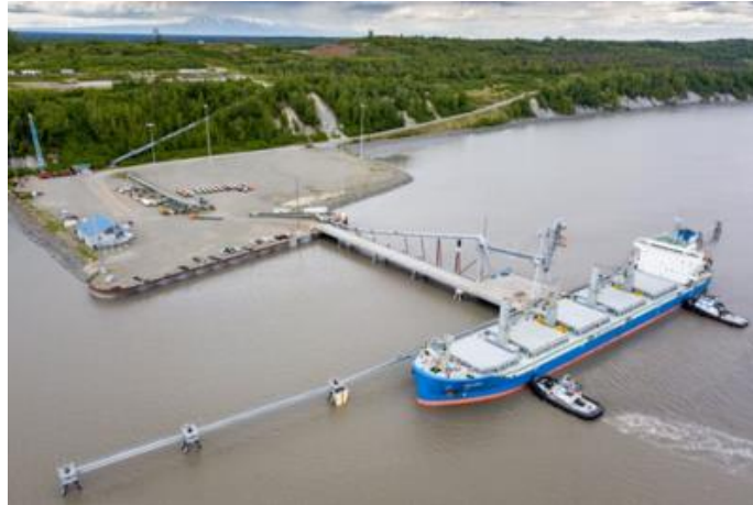
Figure 1 Port MacKenzie Dock and Berth
