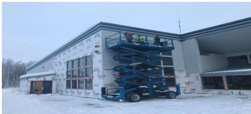
Above Photo: Siding Removed to Prepare for New Library Construction
