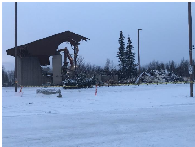
Above Photo: Demolition of Houston Middle School
