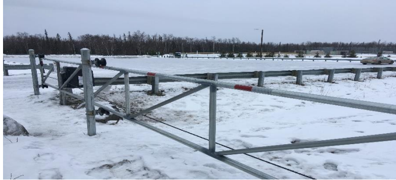
Above Photo: New East Parking Lot Gate Installed
