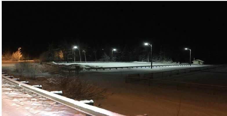
Above Photo: Alcantra West Parking Lot – four new lighting poles installed
