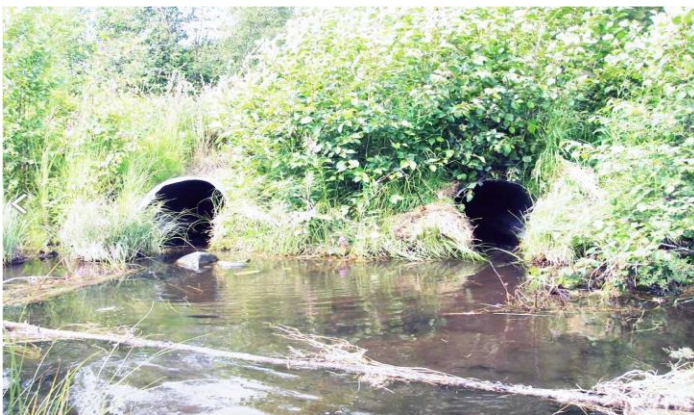
Above Photo: Rubacaba Road at O’Brien Creek
