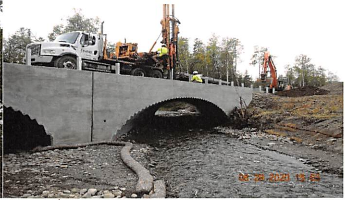
Cottonwood Creek Fish Passage.
