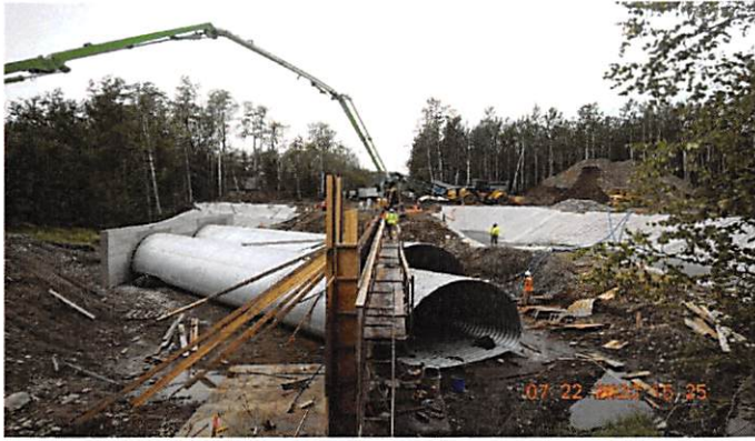
Cottonwood Creek Fish Passage.
