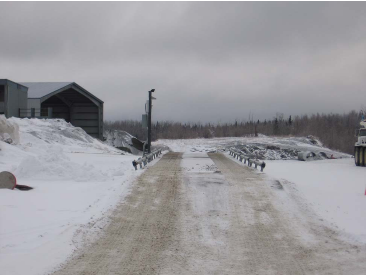
Figure 5- Commercial Scale, Looking South From On Ramp (self serve weigh-in panel on left)
