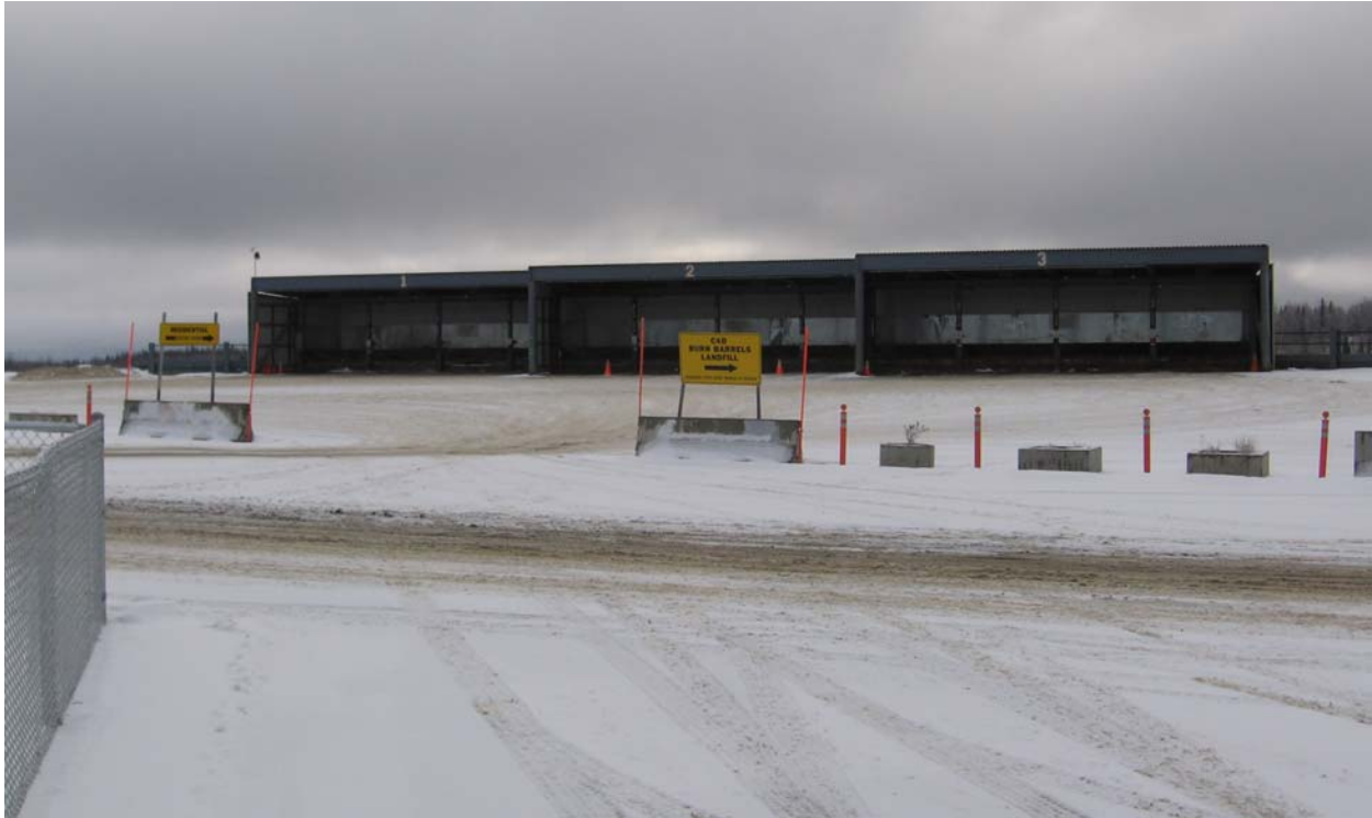
Figure 10- Stage 2, Dumping Area, 12 Stalls in 3 Groups
