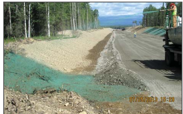
Seeding new embankment along Segment 6 in July 2013.
