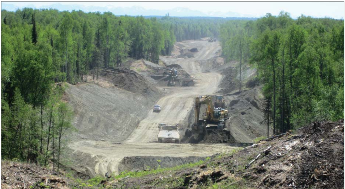
Segment 3 grade work north of W. Susitna Parkway mid-summer 2013.
