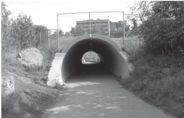
Coastal Trail Culvert/Pedestrian Crossing
