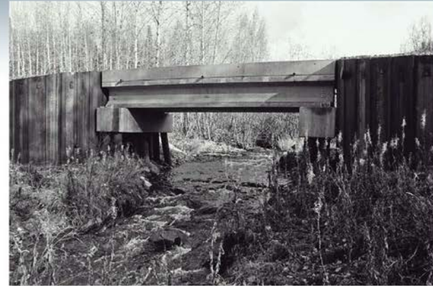
One-Span Multi-Purpose Crossing
