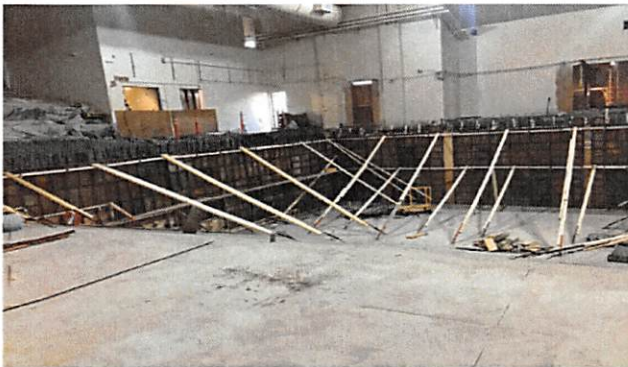
Palmer Pool deep-ended formed walls.
