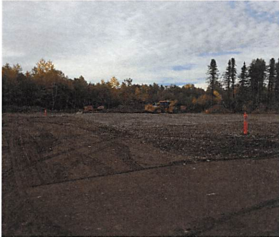
Site Work at Station 11-9
