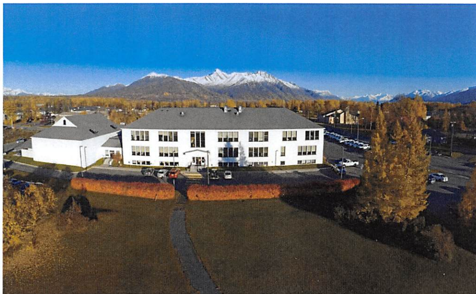
Matanuska-Susitna Borough Administration Building
