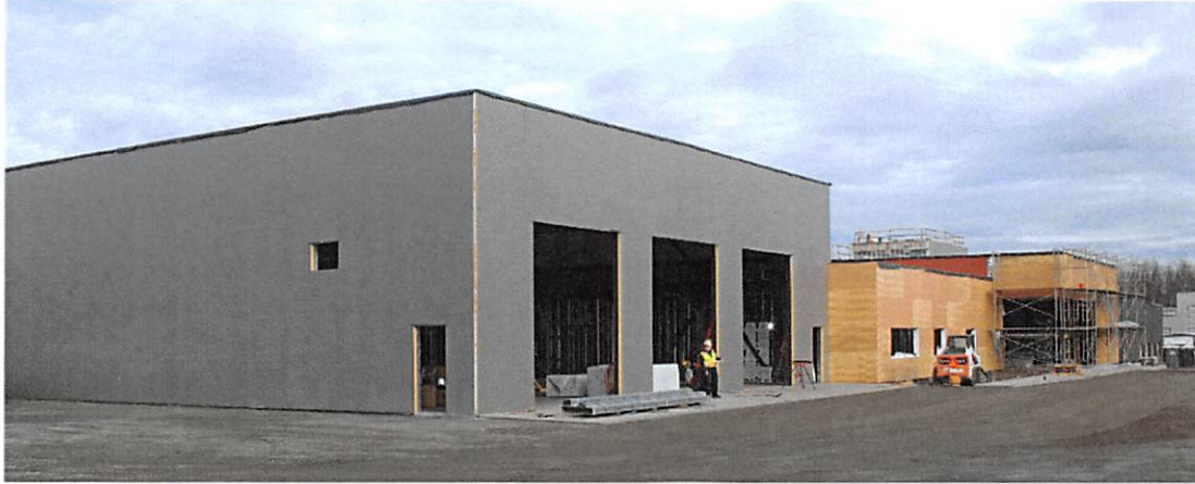
Above: Station 6-2 Construction in progress
