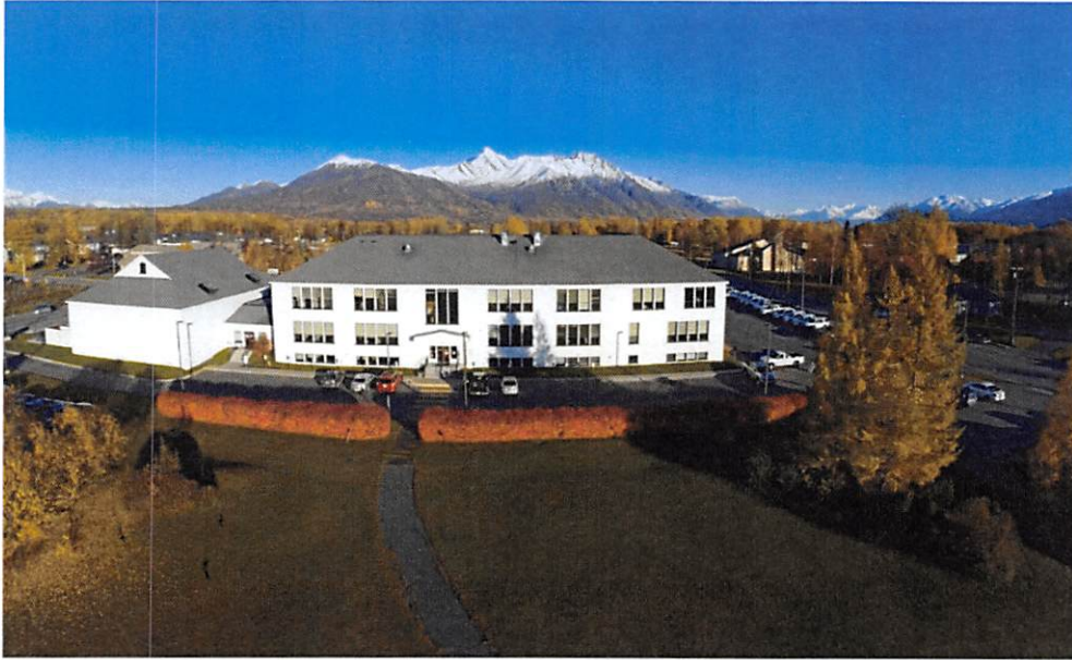
Matanuska-Susitna Borough Administration Building (Photo by: Stefan Hinman)
