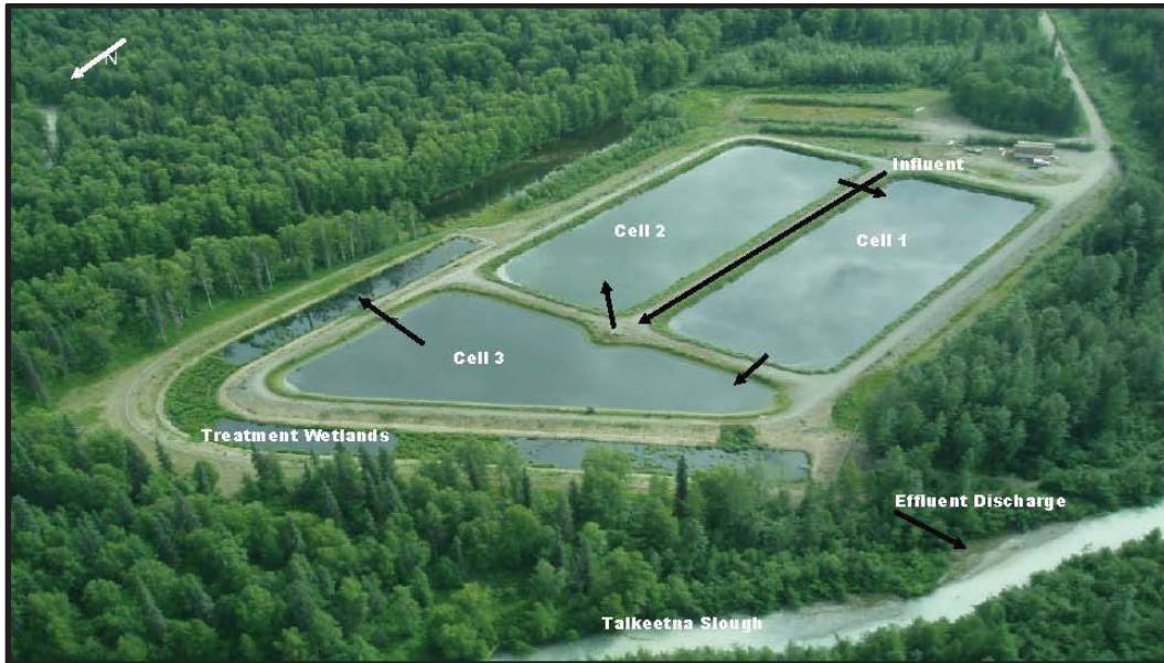
Figure 2: Existing Talkeetna Wastewater Treatment Facility (Photo Taken June 2007)
