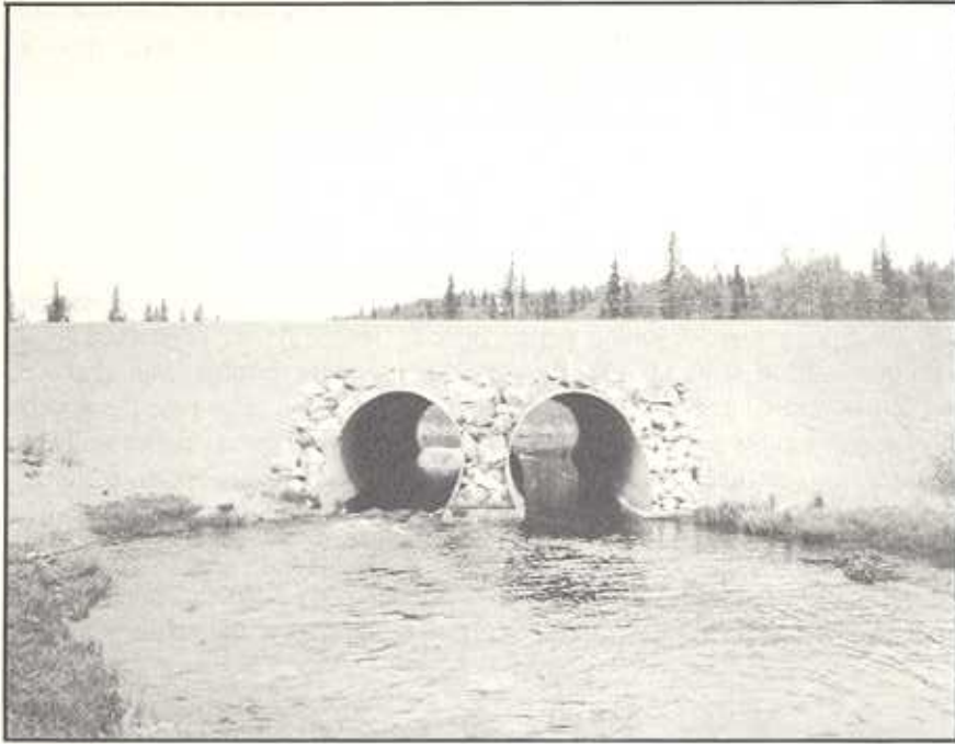
Culverts in 196-Mile Creek at Parks Highway crossing.
