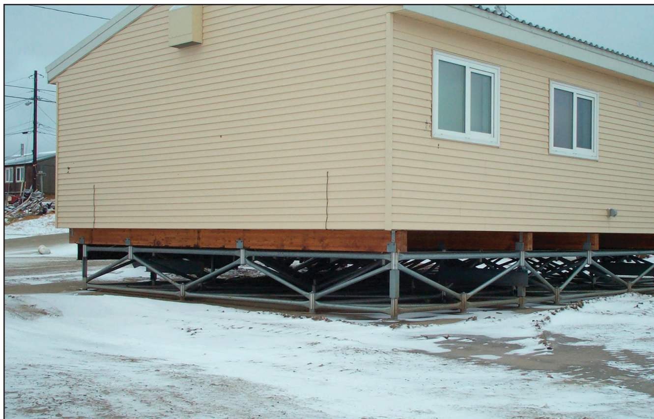
Shishmaref house on Triodetic foundation
