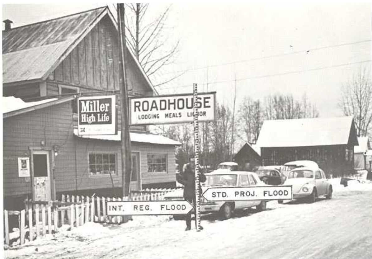
FUTURE FLOOD HEIGHTS AT THE ROADHOUSE ON THE MAIN STREET OF TALKEETNA FIGURE 7
