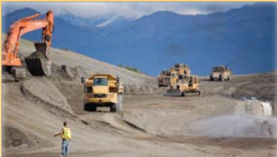
Photos: the ship, the deepest draft vessel ever in Upper Cook Inlet at Port MacKenzie; Above: 2010 haul road and rail loop construction at Port Mac moved 1.9 million cubic yards of dirt.
