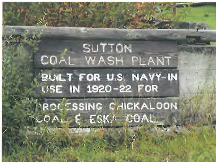
Sutton Coal Wash Plant Sign from http://alpinehistoricalpark.org
