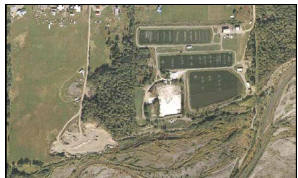
Aerial view of Palmer Wastewater Treatment Plant
