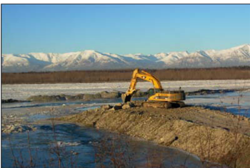
Construction of Dike #5 in Circle View Subdivision.
