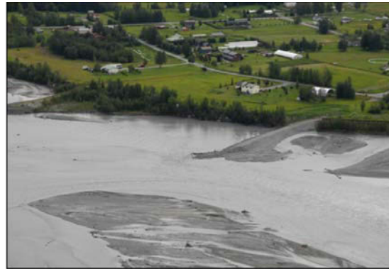
Circle View Subdivision in Butte has a concentration of five finger dikes, like the one shown above, to protect against erosion.
